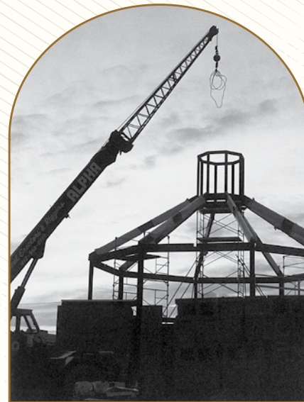
The steel structure forms the foundation for the Magdalen Chapel. (1989)
