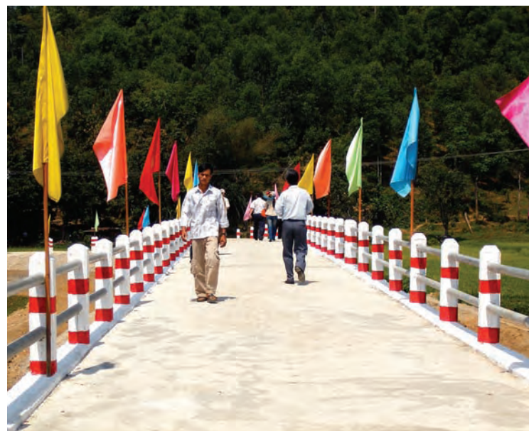
The Hoi Yen bridge connects two villages (Nam Yen and An Dinh) and allows children a safe passage to school during the rainy season.
