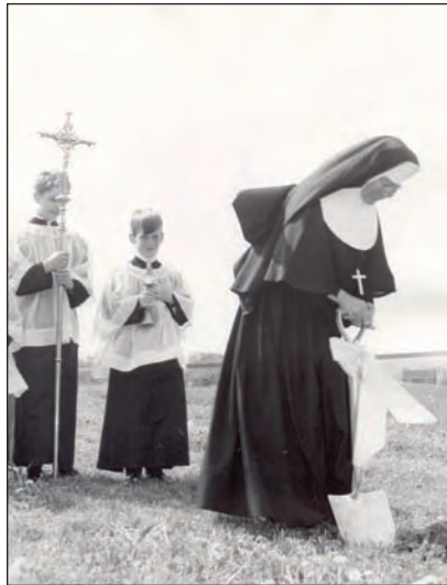
Mother Mary Dominic Obringer, CDP, Provincial Superior, Sisters of Divine Providence, breaks ground for the Wright Library in 1966.
